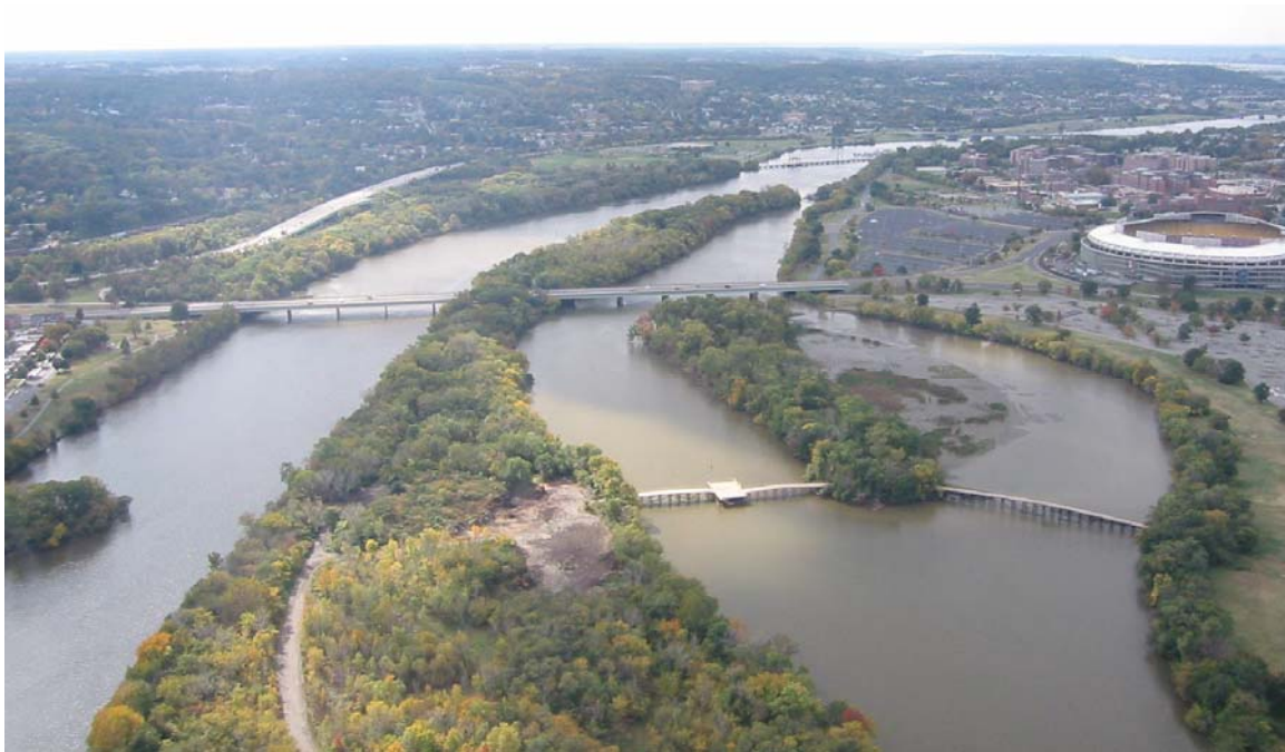
An aerial photo of the Anacostia River showing Kingman and Heritage Islands
