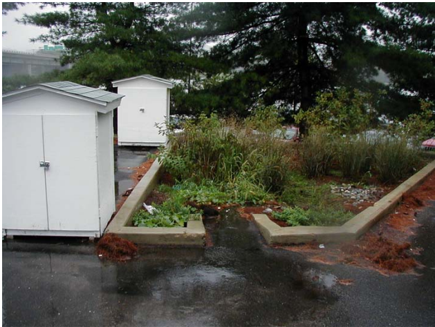
A rain garden filtering pollutants from a parking lot at the Washington Navy Yard.
